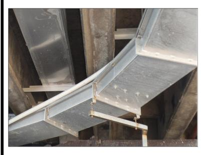
• M.A. Smith Engineering (NSW) Pty Ltd have manufactured special purpose custom designed cable trays for specific installations.
